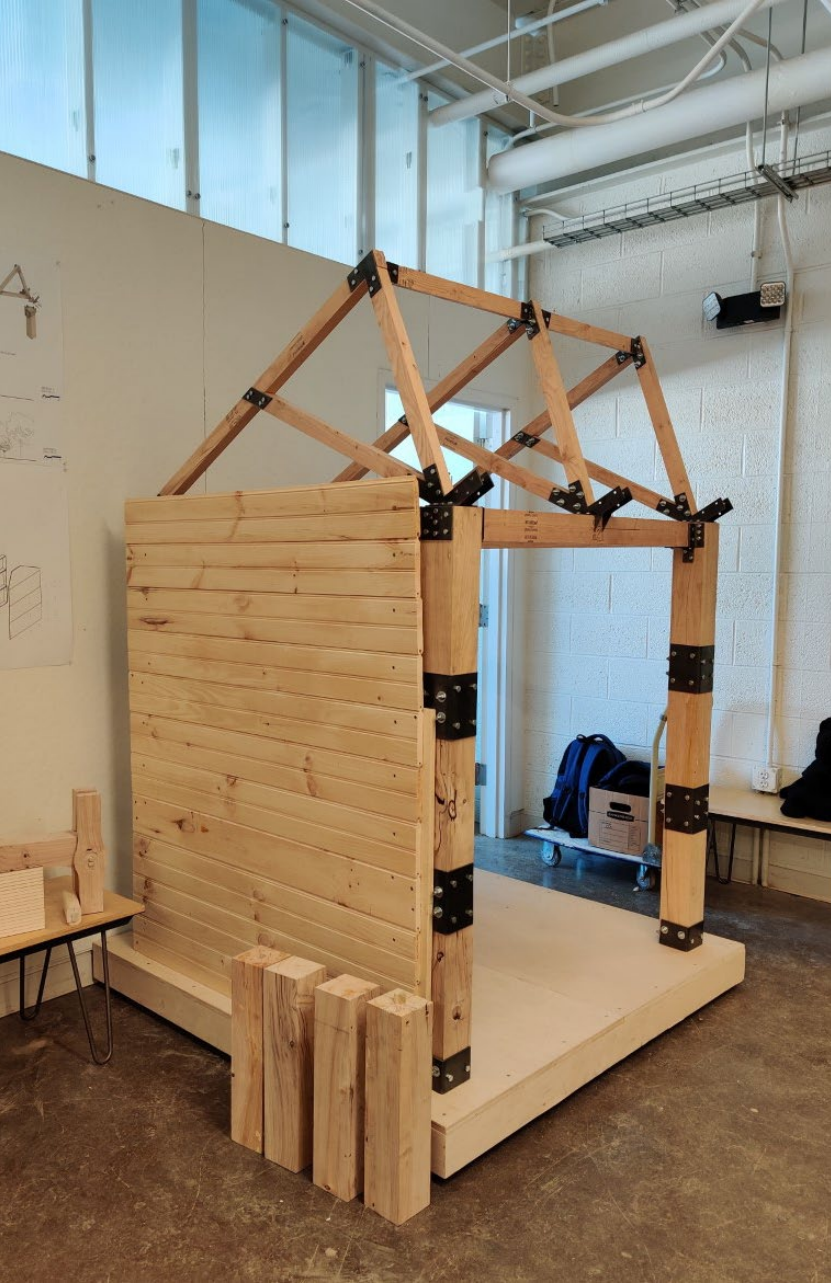
Left- A prototype of the first structure and shell system, Right: the second structure+shell system made out of reused elements obtained from the first system. Credit: Students in DfD Studio, John Mark Nachbar, Ana Alarcon, Raymond Jacobson.
