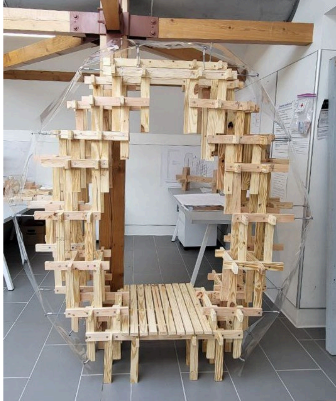
Left- A prototype of the first structure and shell system, Right: the second structure+shell system made out of reused elements obtained from the first system. Credit: Students in DfD Studio, John Mark Nachbar, Ana Alarcon, Raymond Jacobson.
